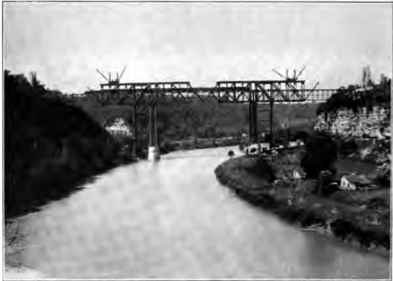
A FAMOUS CANTILEVER RAPIDLY DISAPPEARING — THE SUBSTITUTION OF A NEW KENTUCKY RIVER BRIDGE FOR THE OLD, ON THE QUEEN & CRESCENT SYSTEM
